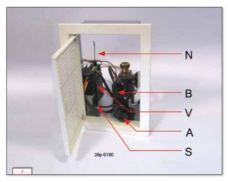
!Caution - Do not place the antenna (N) too close to the ignition cable and/or metal parts: make sure the antenna is pointing upwards (for the correct position, see fig. 1);
